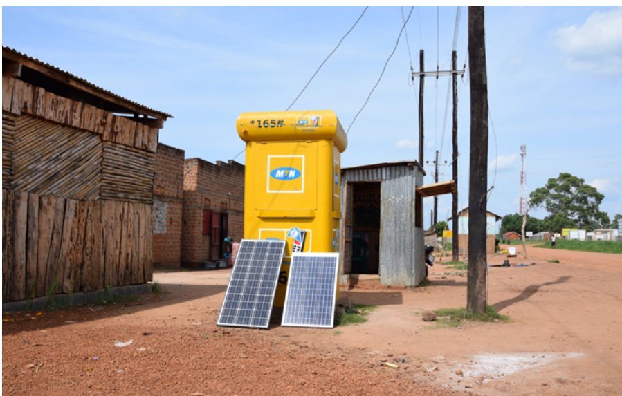
Solar (PV) panels leaning against a telecom provider booth next to power lines forming part of the grid.
