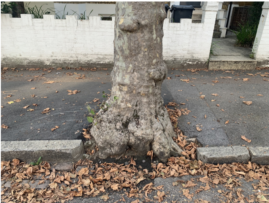
A curb is removed to make space for an expanding tree, London. Photo: Aaron Bradshaw, 2023.
