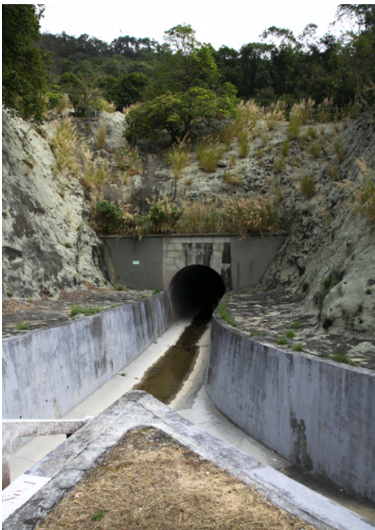
Two catchwaters divert into a tunnel that distributes the water to the reservoir across a mountain ridge. Artificially engineered slopes of concrete protect the catchment from erosion.
