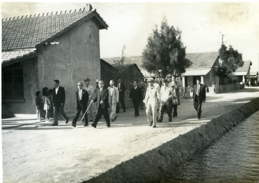
SWH housing at Budai Saltworks.
