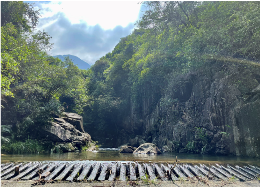
Concrete water grate intake in the upper reaches of the Tung Chung River's western stream.
