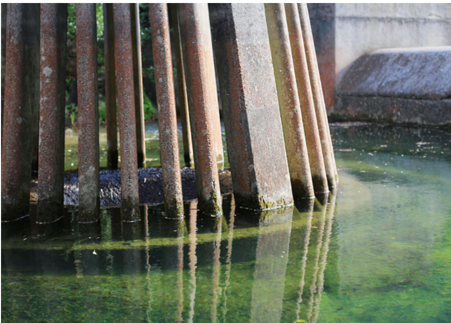
Detail of a prefabricated conical structure with a water intake set inside.
